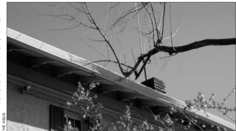
Figure 87 This branch is a virtual highway to the roof for squirrels. After repeated invasions of the building, the branch was finally trimmed back and squirrel traffic rerouted to nearby trees.
