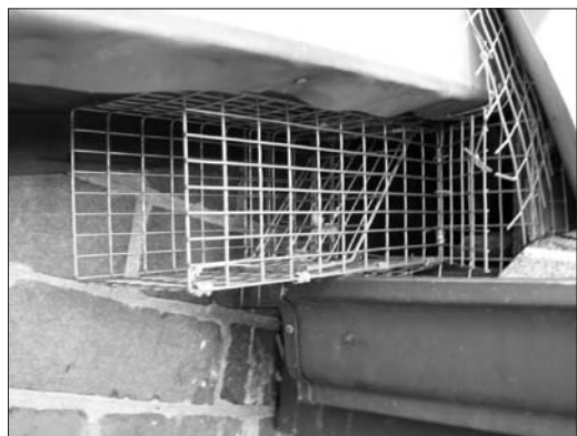
Figure 90 This commercially made one-way door is set where a family of squirrels has been entering and leaving a house. The young are old enough to be mobile, and all will be safely evicted using this device and prevented from getting back in.
